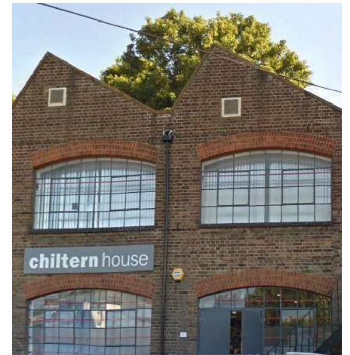
▲ Fig 1.4 | Chiltern House [Industrial Building]
